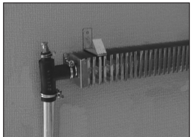
Convector and hose connection with bleed nipple.
