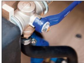
Direct drain – waste water bypass tank (standard in Imperial)
