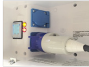
Electricity meter in the electrical box
