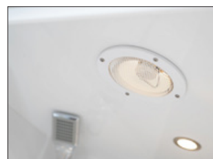
Ventilator in de badkamer (TDL)
