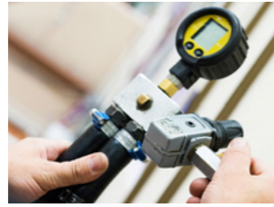
GAS SYSTEM The gas system is pressure tested.
