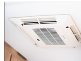
Klimaanlegg bodel Fresh Jet FJ2200 (standard Imperial)
